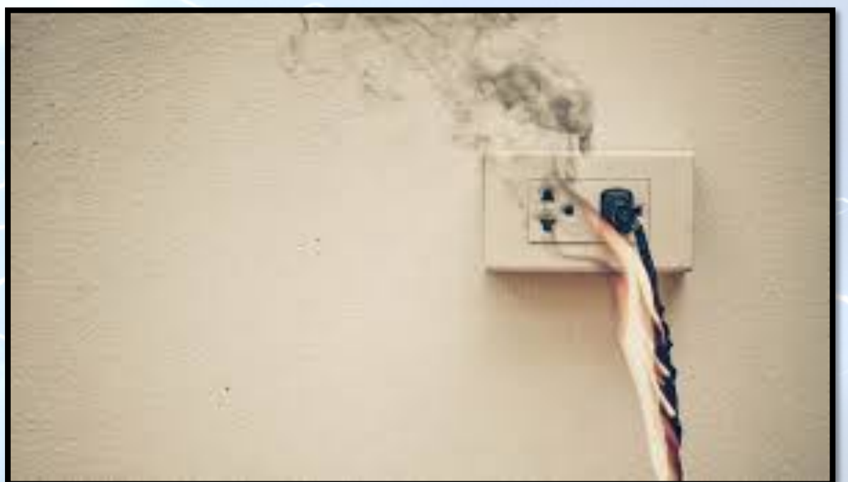
A power outlet that has been damaged from a power surge. 2
